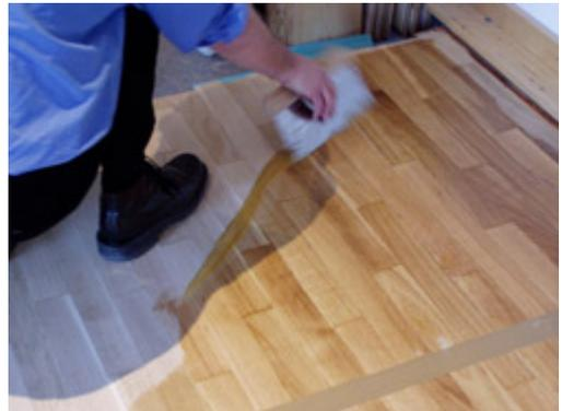
After two coats the floor should be fully finished. Leave for about a week before giving any heavy wear, moving heavy furniture etc. For the best results buff down with liquid wax cleaner two weeks after finishing.
