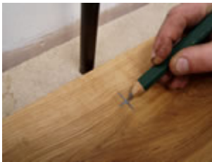
1. Carefully mark the position of the pipe.
