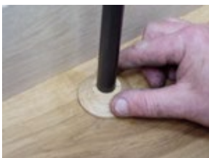
7. Fit a pipe cover in a matching timber.
