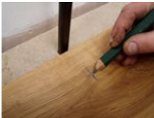
1. Carefully mark the position of the pipe.
