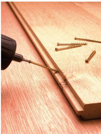
Tongue-Tite™ screws have an advantage over flooring nails in that they are self-piloting and countersinking, and do not require specialist equipment for use. The screws nip the boards together tightly, and have the benefit of being easier to remove and reposition, if required.
