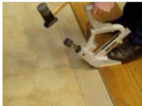
Even more popular are the specially designed Tongue-Tite™ flooring screws which are fixed through the tongue joint (at an angle of approx. 30 degrees) using an ordinary drill or
