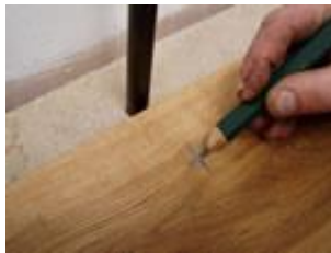
1. Carefully mark the position of the pipe.
