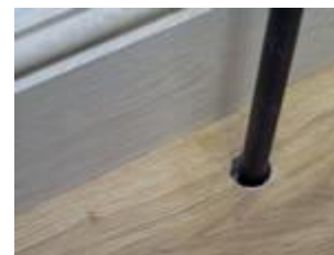
6. Slide back over the pipe and glue wedge in place.
