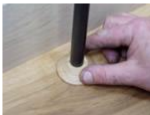
7. Fit a pipe cover in a matching timber.
